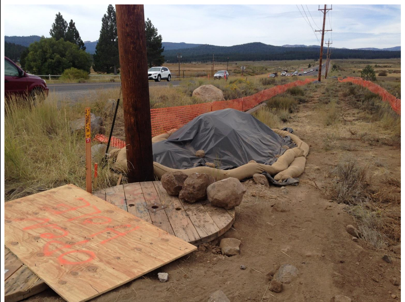
Photo 1: Topsoil salvage piles covered with BMPs installed (straw wattles), consistent with APM-BIO-23. Excavated pole holes covered to prevent wildlife from entering holes.
